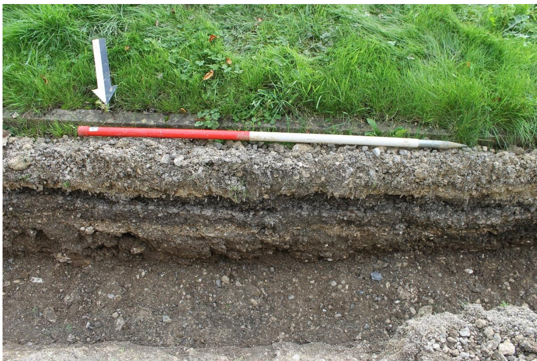
Plate 2 Water pipe trench through gravel path (1000). North-facing section. 0.5m scale units.
