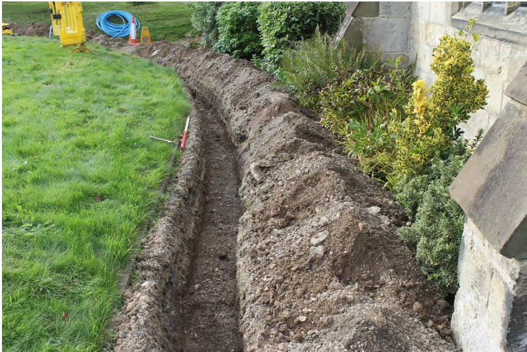
Plate 3 Water pipe trenching, south side of the church. View looking west. 0.5m scale units.
