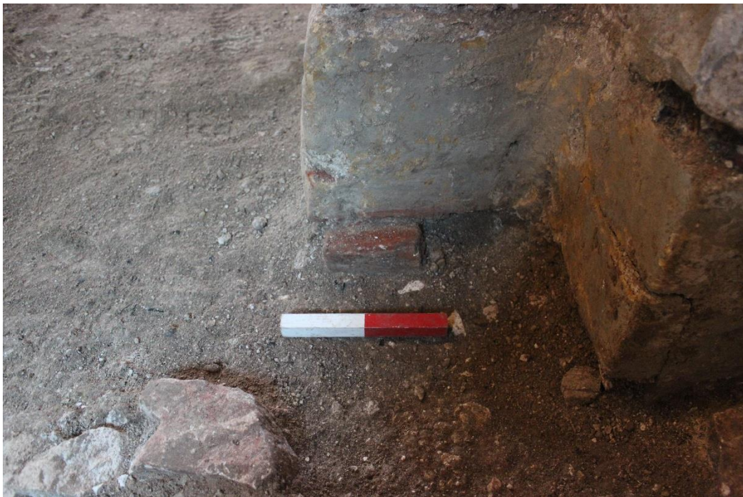
Plate 20 Brick repair [3011] below extant archway of nave. View looking south. 0.1m scale units.
