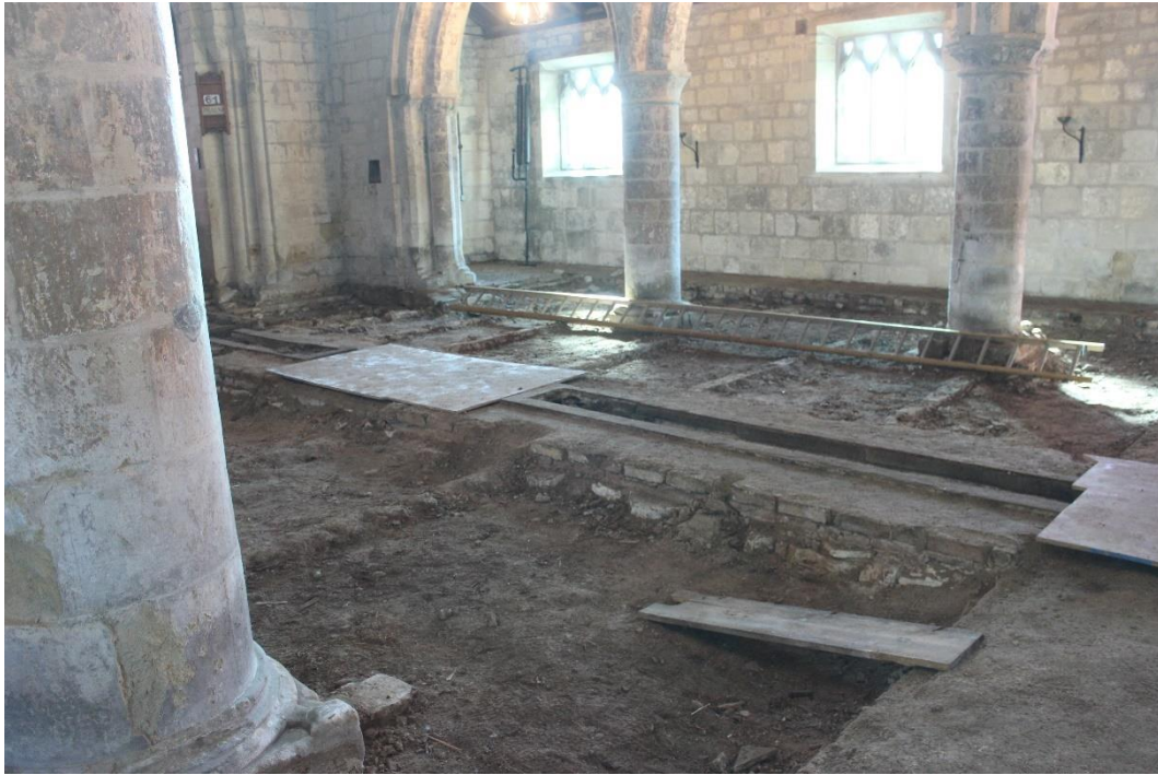
Plate 31 Central heating channel [3027], abutted by bricks 3000 and stone 3001. View looking south-east.
