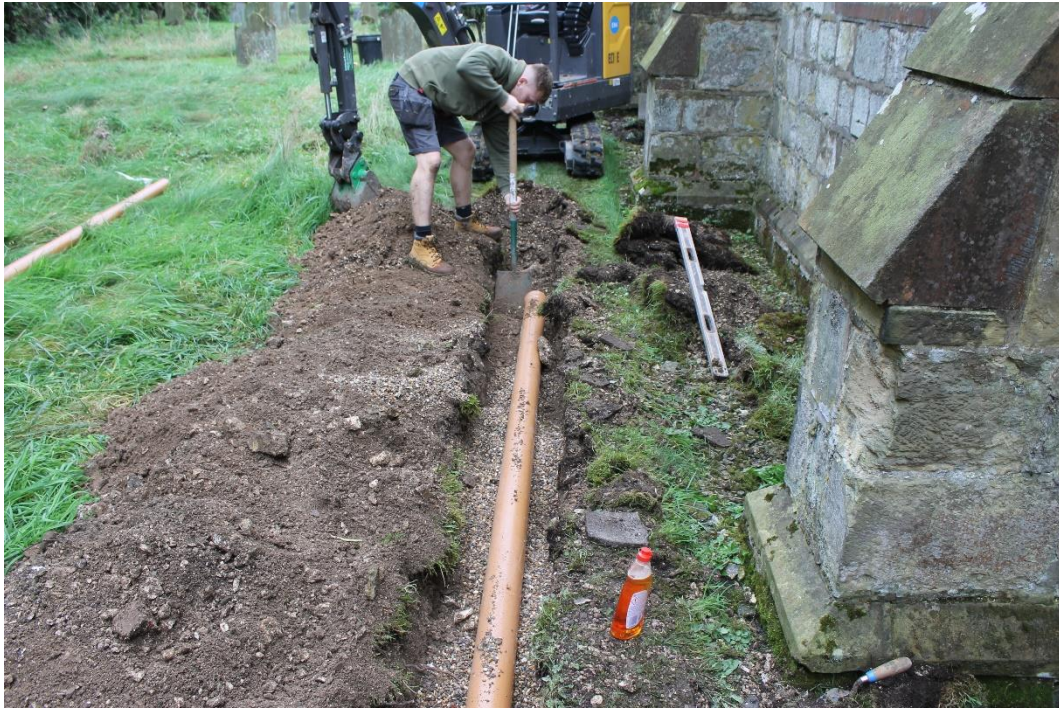
Plate 7 Drainage trenching on north side of church. View looking east.
