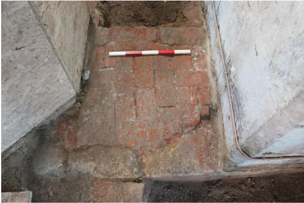
Plate 33 Brick surface [3022] exposed below font. View looking west. 0.1m scale units.
